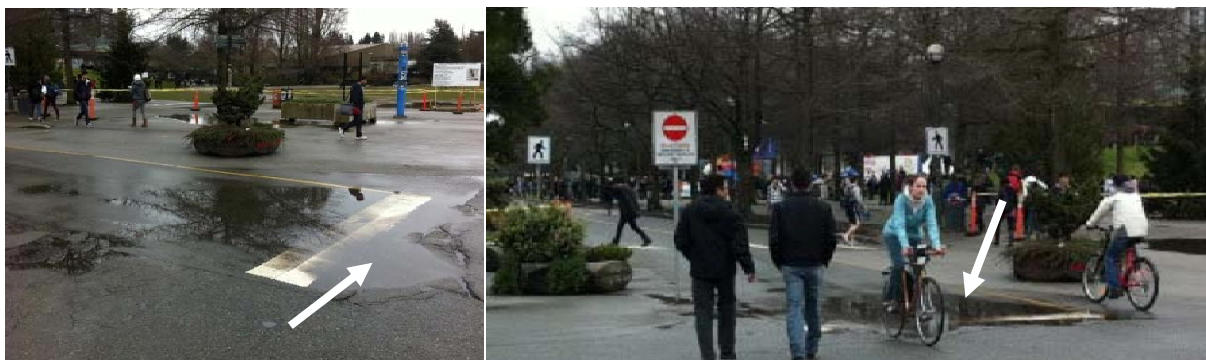
Figure 6 – Photos showing the common occurrence of temporary flooding at and around the New SUB location, just after a few hours of moderate rainfall as indicated by the arrows (photos by Peter Woo, 2011).
