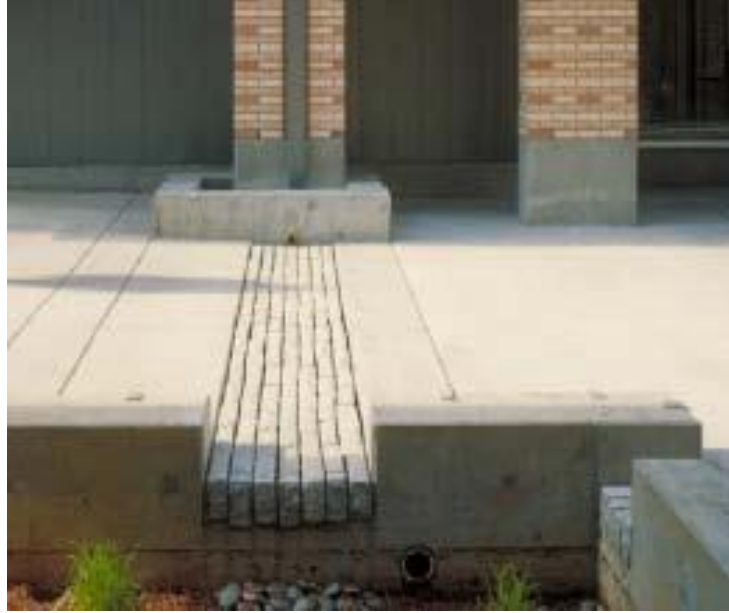
Figure 2 - Drainage to Rain Garden (UBC SUB Team and Associate, 2010)
